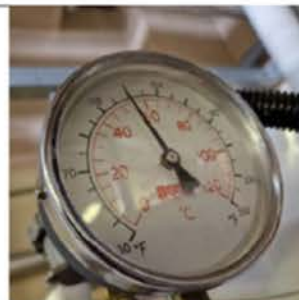
Hot Water Flow Temperature gauge – Reading 55°C
