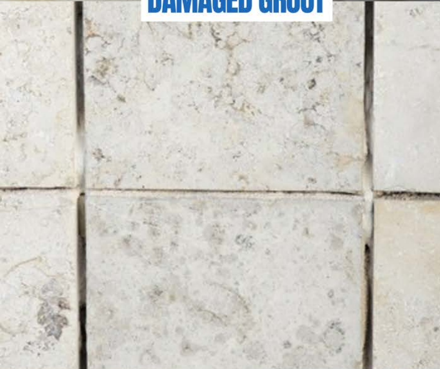
DAMAGED GROUT
